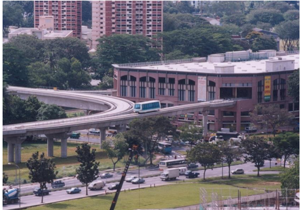
Project: LRT Depot & Mall Bukit Panjang, Singapore
